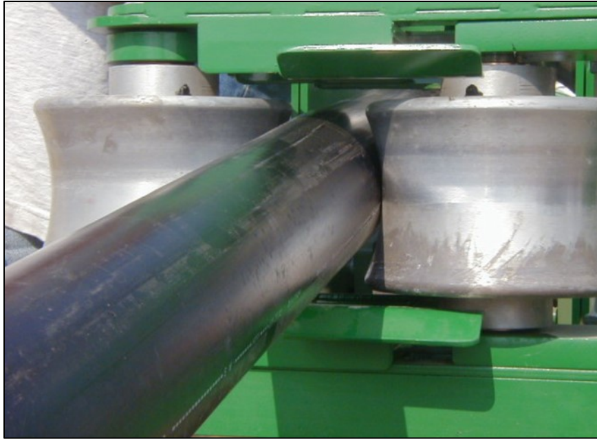
Figure 16: HDPE coiled conduit passing through a re-rounding device (close-up)
