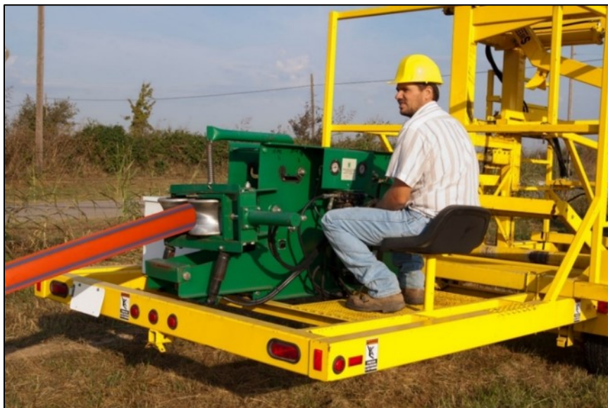
Figure 15: Nominal 6 in. coiled conduit being pulled through a re-rounding device
